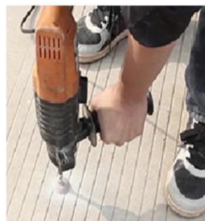
3.Use an electric drill to punch holes
